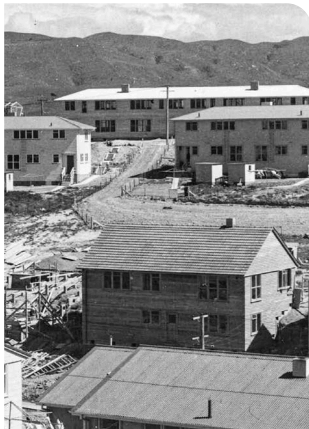
Houses on Champion Street, Cannons Creek, being built in the 1960s
